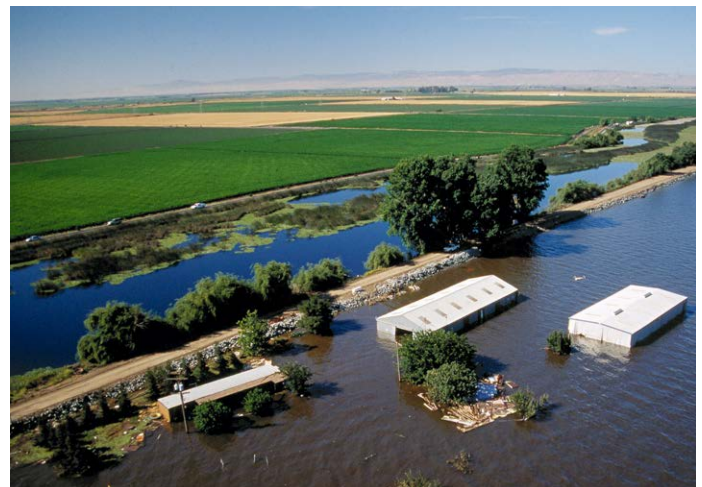
Photo of flooding caused by the 2004 Jones Tract levee breach. Photo credit: California Department of Water Resources.
