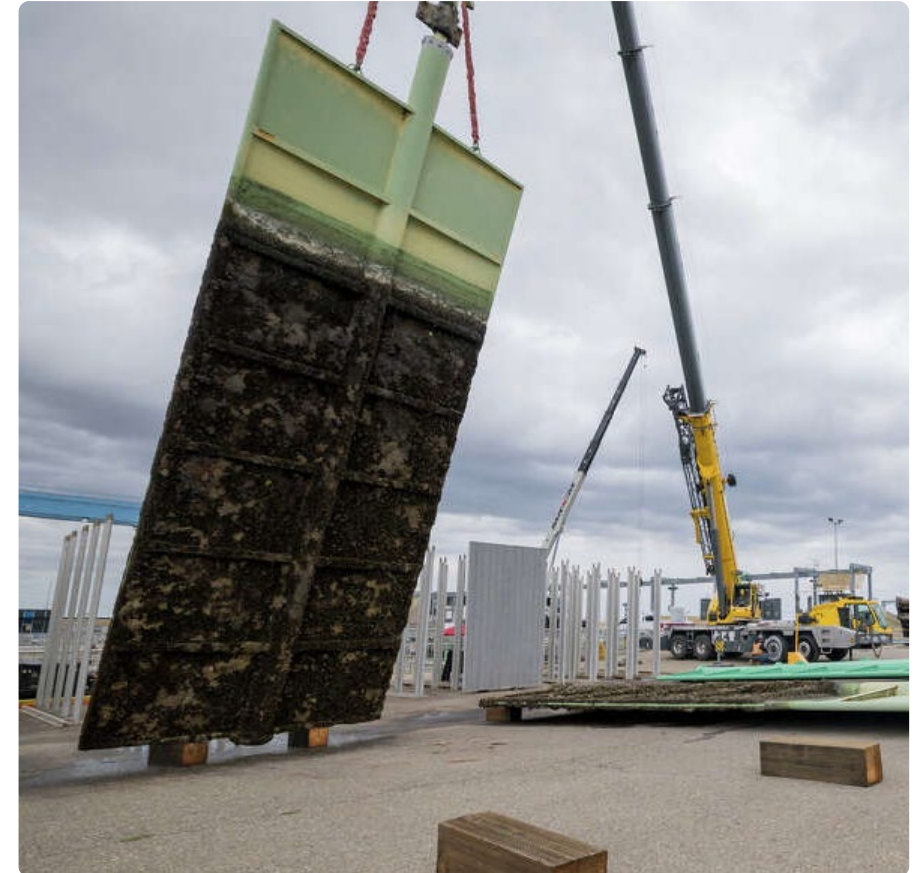
Mussel-covered wing gate replacement during annual maintenance at Skinner Fish Facility on May 4, 2026 (DAC Appeal, p. 10)
