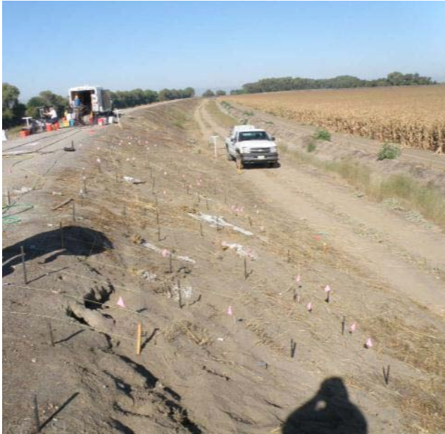
Levee site pre excavation
