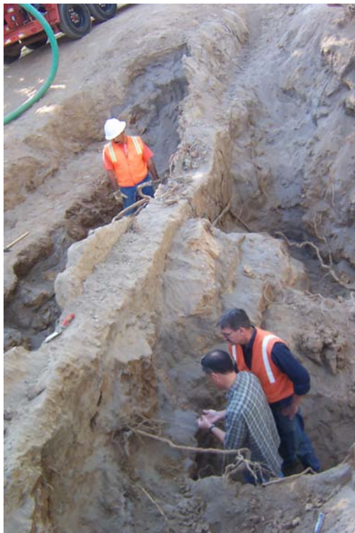
Exposed slurry wall (Pocket area levee)
