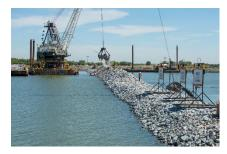
Emergency drought barriers were first placed during the 1976-77 drought in six places in the Delta to quell salinity intrusion (DWR 2015). A barrier was used again in 2015 and 2021 in False River to stop saline water from entering Franks Tract which is located near waterways used to convey fresh water to the CVP and SWP (see Emergency Drought Salinity Barrier fact sheet for more information).
