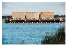
The use of operable gates on waterways that are used for freshwater conveyance can reduce salinity intrusion by redirecting the flow of fresh water. The Delta Cross-Channel (DCC) is a constructed channel with two operable gates that can divert water from the lower Sacramento River into the Central Delta via the Mokelumne River. The operation of the DCC redirects the flow of fresh water into
