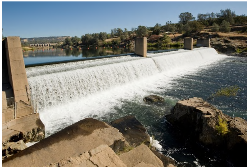
Salmon diversion dam on Feather River (source: iStock)
