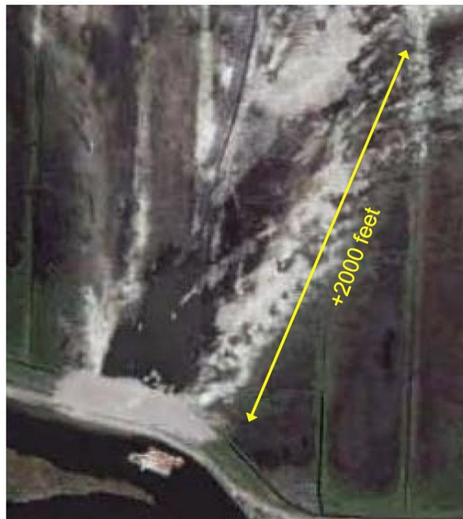
1 Scour Hole from Jones Tract Levee Failure Source: East Bay MUD
