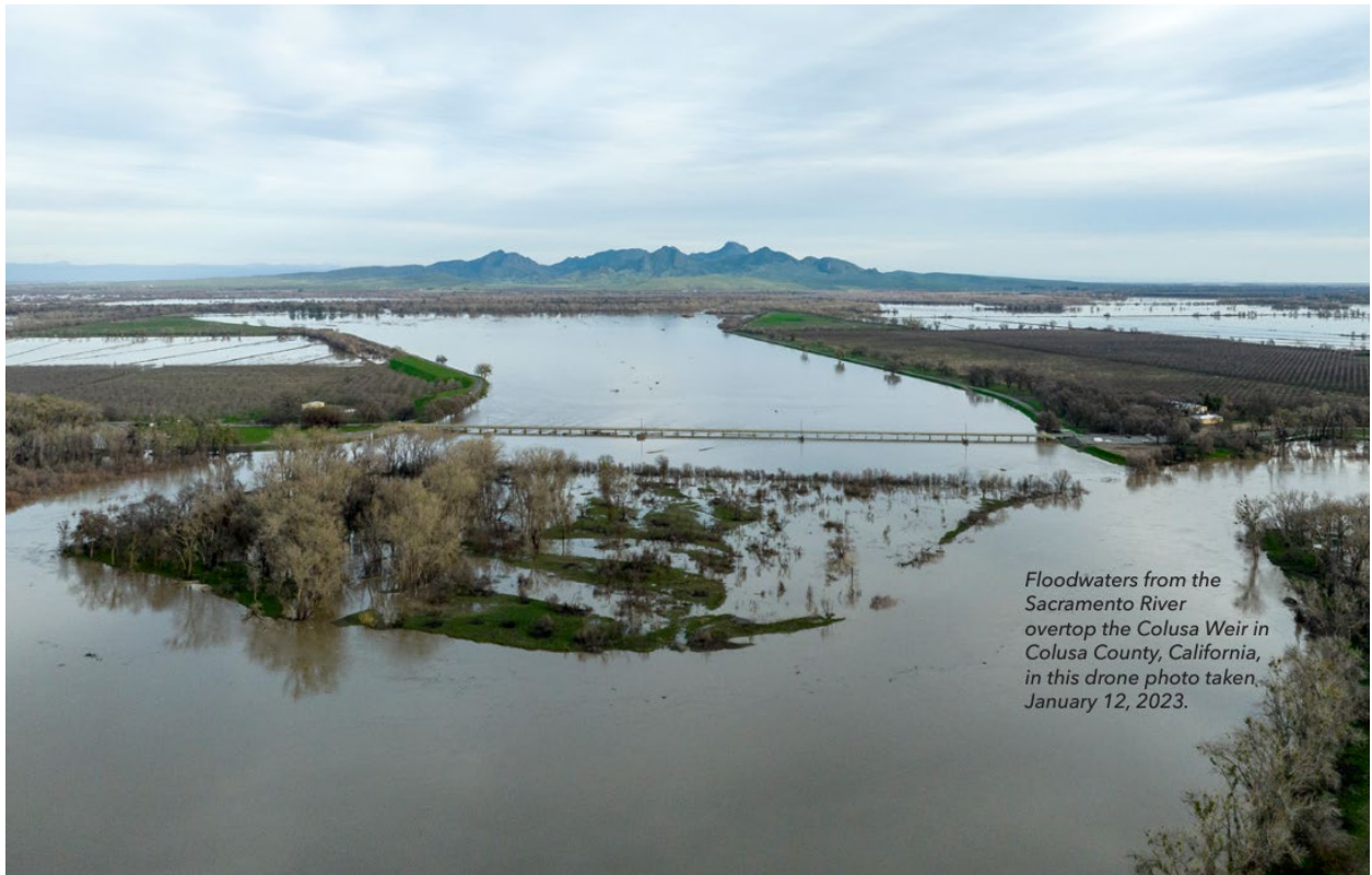
Figure 2 - Colusa Weir is overtopped by Sacramento River on January 12, 2023. Central Valley Flood Protection Plan Update 2022 / January 2023.
